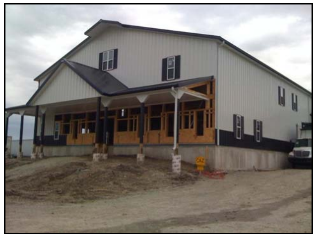
Began Construction of a new facility at the farm.
